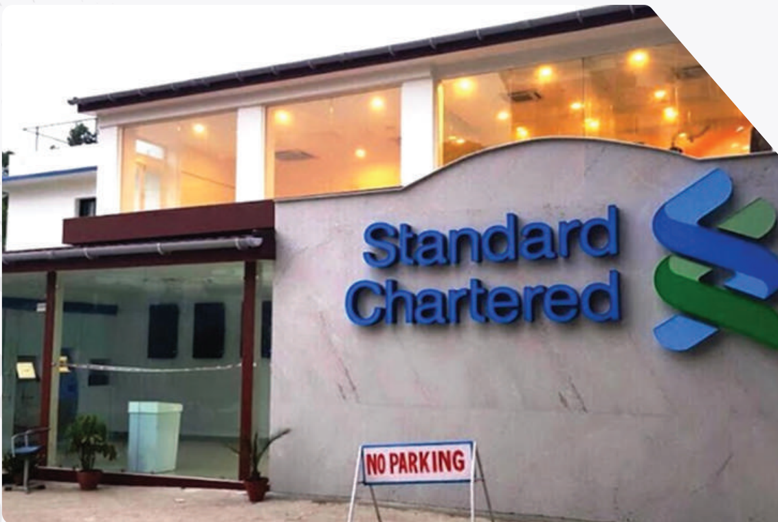
Project: Seismic Retrofitting Works at Standard Chartered Bank, Lazimpat Branch, Nepal.
