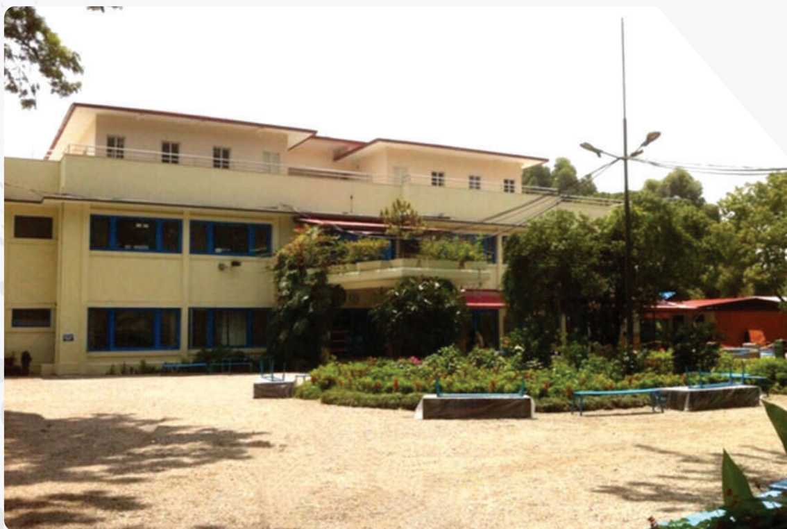
Project: Seismic Retrofitting Works at The British School, Jhamsikhel, Lalitpur, Nepal.
