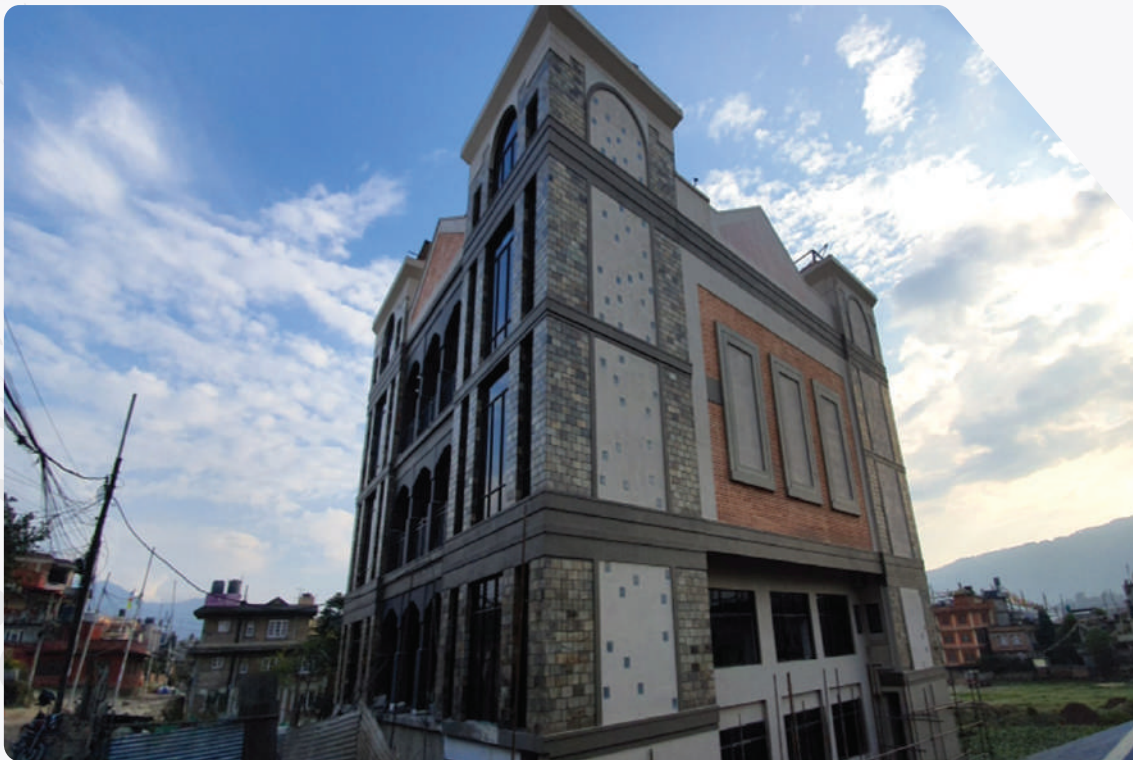
Project: Crossway Church Building, Ekantakuna, Lalitpur
