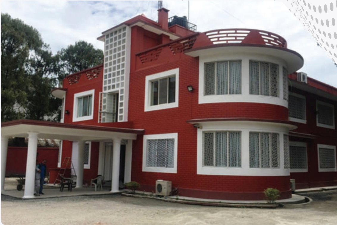
Project: Strengthening of the External walls and Securing of the internal Partition walls of French Embassy Chancery Building, Lazimpat, Kathmandu, Nepal.
