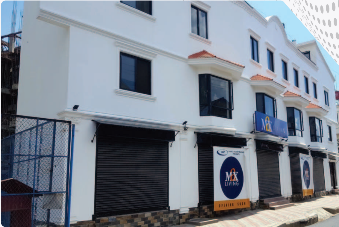
Project: Construction of Commercial Building for Mr. Sarad Rana
