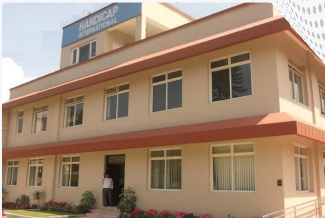
Project: Retrofitting & Interior Construction Works of Office Building, Director's Residence & Guest Block, Maharajgunj, Kathmandu.
